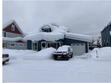
(D) Corncicing and snow accumulation around dormers
