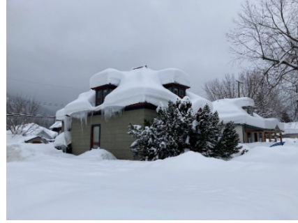
(B) Snow accumulation between dormers
