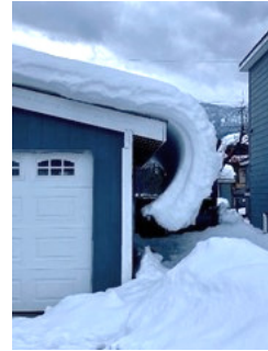
(F) Sliding snow causing corncicing
