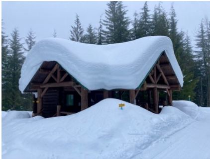
(E) Snow accumulation in a roof valley
