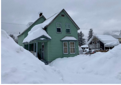
(A) Sliding snow causing accumulation on low roof
